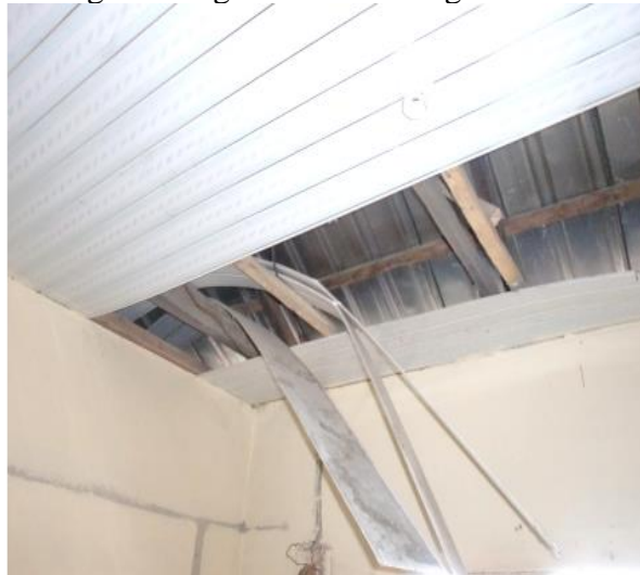
Figure A2. Building showing caved-in ceiling in one of the communities
