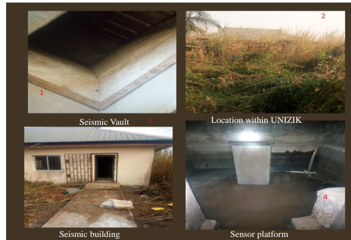
Fig. 1.3: Seismic station in Awka constructed in 2008 showing building, vault of about 4 meters deep, and platform for the sensor.
