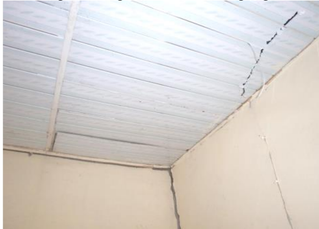
Figure A2. Building showing caved-in ceiling in one of the communities
