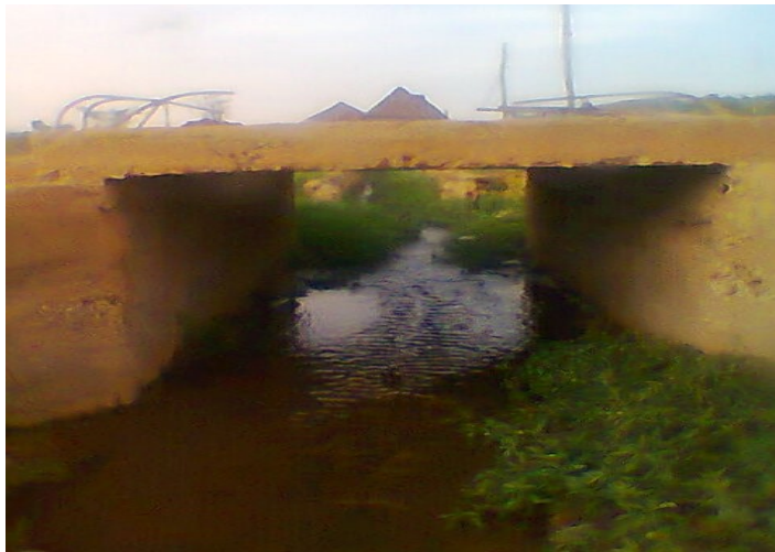
Plate 1: Drainage been covered on top (Source: Field Survey, 2018)
