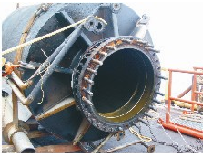
Figure 3: View showing Bottom Area of Burner
