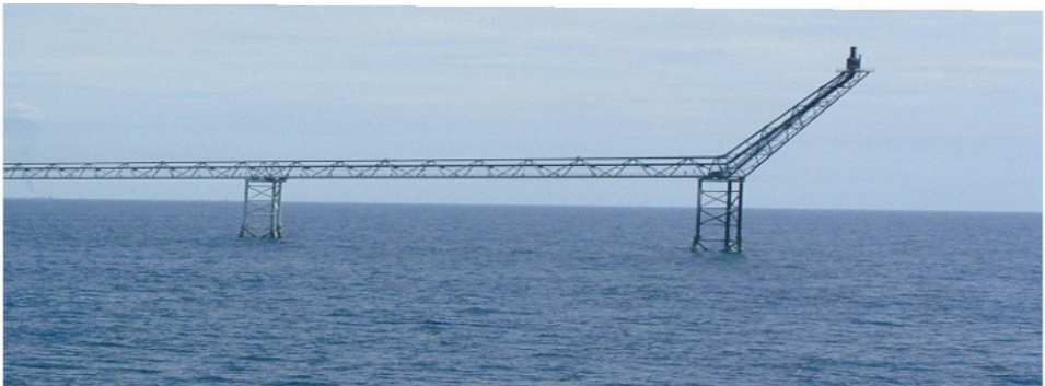
Figure 1: Cryogenic Flare Header / Burner Arrangement
