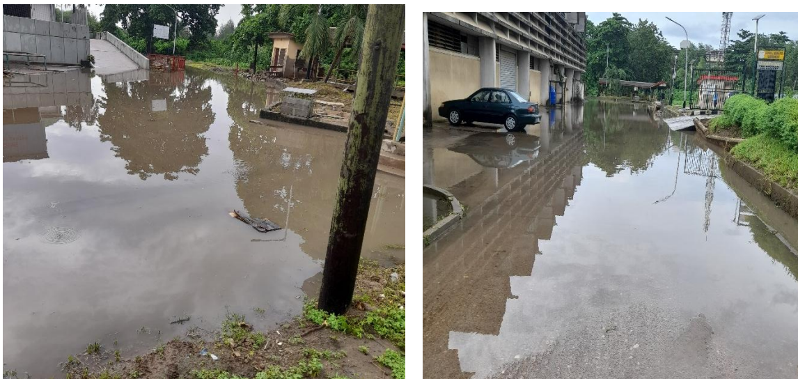
Figure 1: Typical flood along Oduduwa road by Faculty of Engineering workshop after rainfall.
