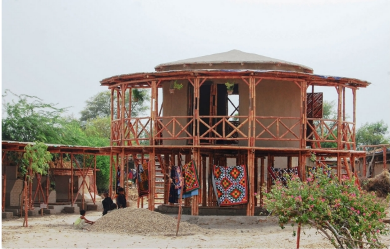
Figure 3: The Green Women's Centre made of prefabricated bamboo modules on stilts, an example of Yasmeen Lari's barefoot architecture
