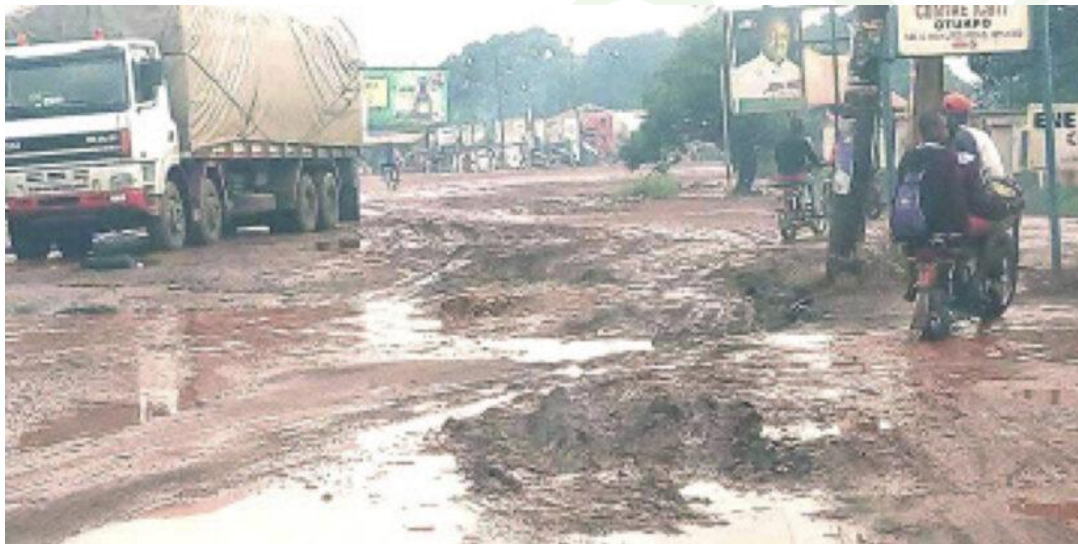
Figure 8: Nigeria bad roads (source: Independent, 2025)
