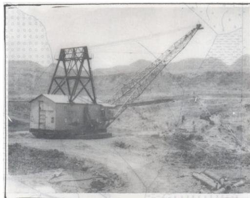
Fig. 7. A dragline for removal of overburden.
