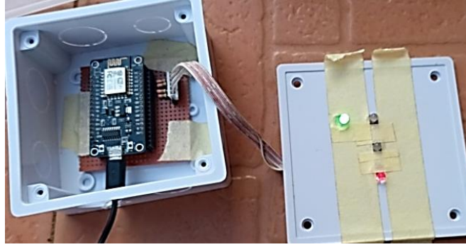
Figure 7c. Hardware access indicator light showing access denial state
